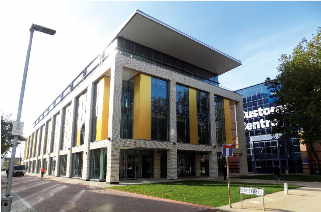
Figure 3.2 Office Building, Centre Square
