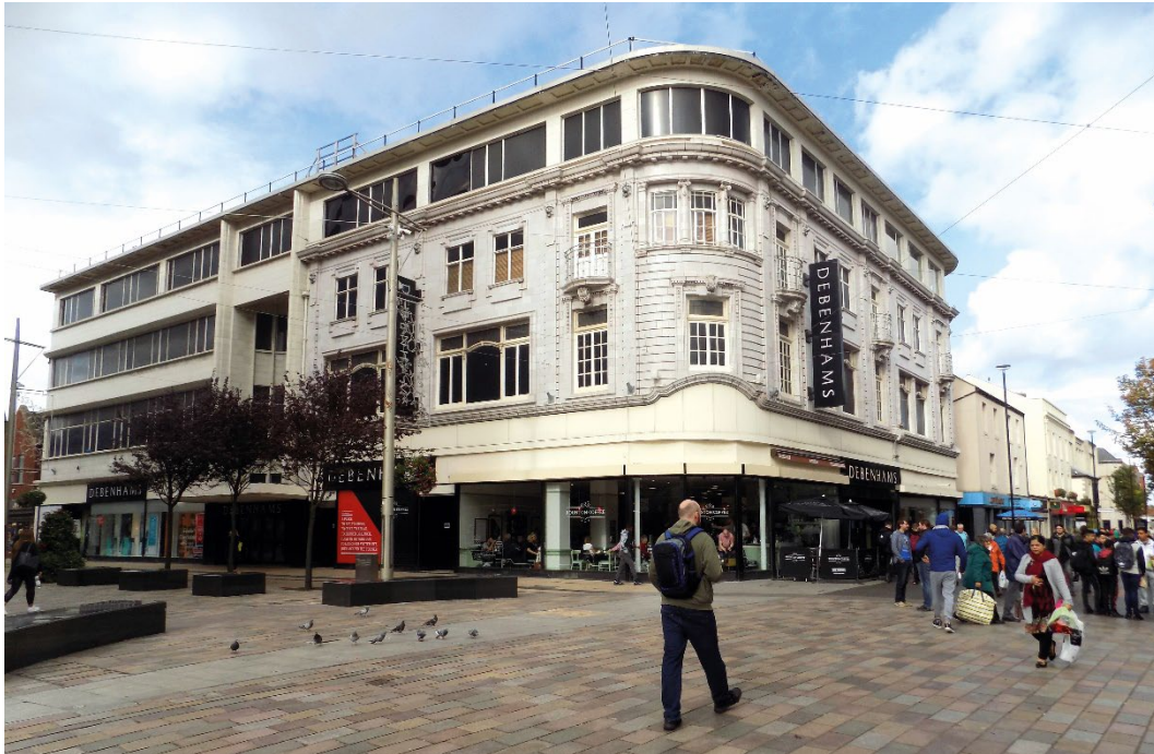
Figure 3.1 Corporation Road/Linthorpe Road
