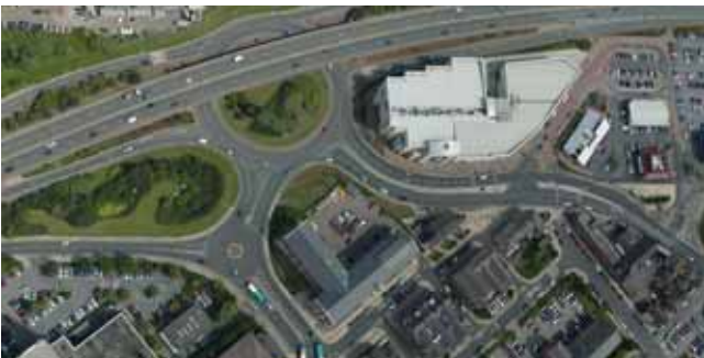
An aerial view of the Marton Road/A66 junction close to Middlesbrough town centre
